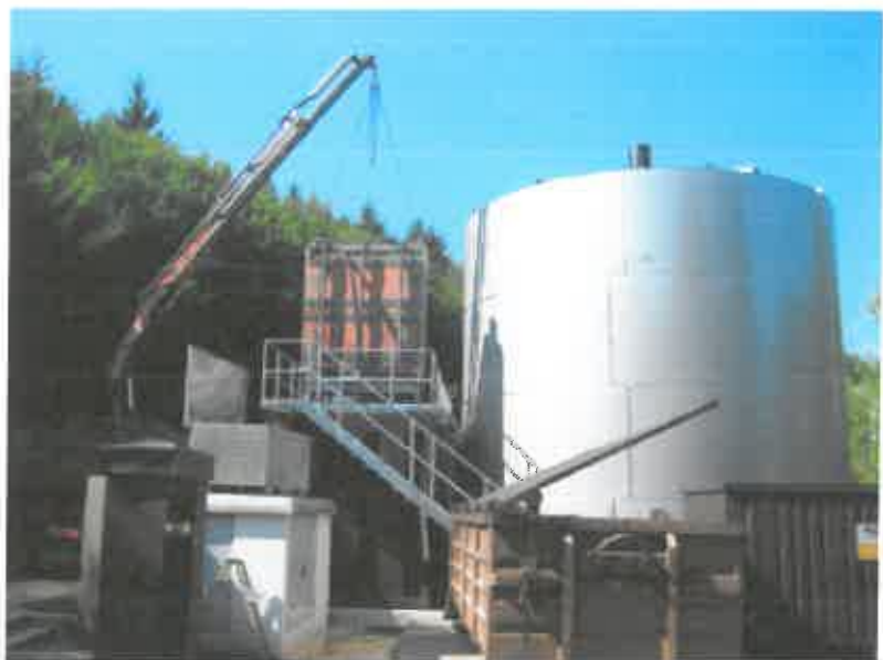
Double-stacked MaxFlow® modules being lifted into tank
